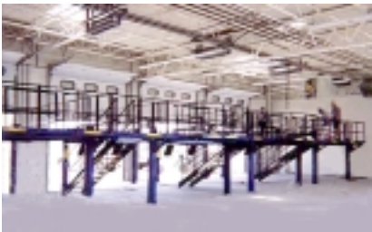
Lube Racks — Mezzanine 4 bay
